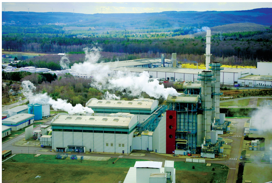
Around the current Émile-Huchet power plant in Saint-Avold, many projects will participate in the economic and industrial relaunch of the territory.
